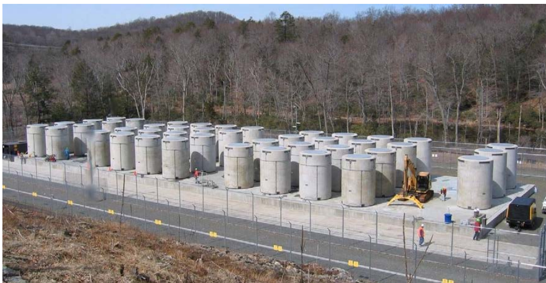
F-10.8-2 Concrete Casks Storage at the Connecticut Yankee Nuclear Power Plant Site
